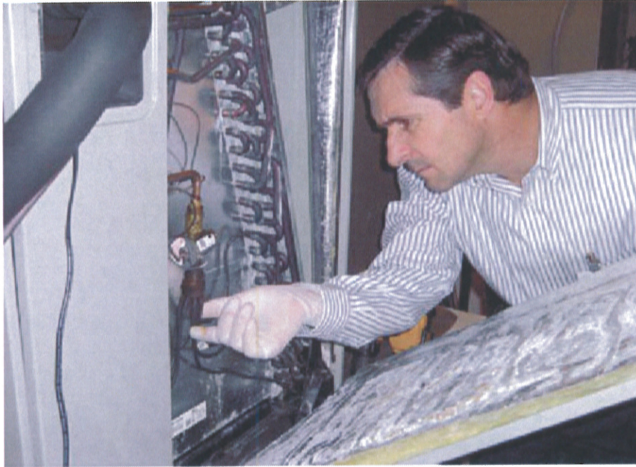
Spiderman Mulholland inspects air conditioning system coils in a Boynton Beach home for signs of toxic Chinese drywall. One sign would be blackened coils.
